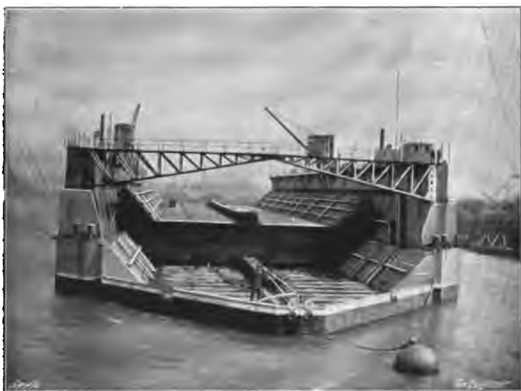
Fig. 515. —Centre Pontoon connected to Dock in Upper Position and lifted Clear of the Water.
